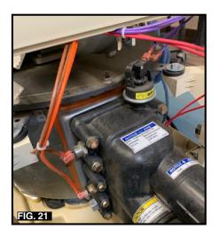
Connect the Water Pressure Switch and AGS switch. The AGS is located on the right side. (Fig. 22).
