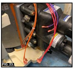
20. Connect the Thermistor sensor and High Limit Switch. *Note: The Thermistor sensor is located at the top of the manifold. The High Limit switch is located at the bottom of the manifold.* (Fig. 24).
