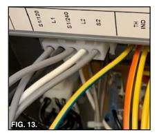
10. Connect S1/240, located on the left side of the 5-pin connector. (Fig. 14).
