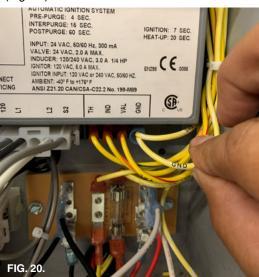
17. Connect the 24 VAC plug at the upper right side as shown in Fig. 21.
