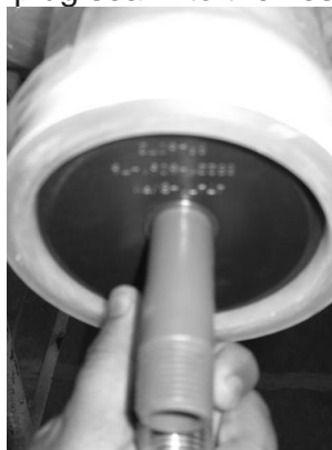
Installation of the End Plug Assembly into the vessel
