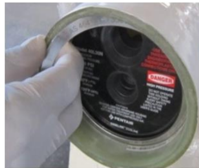
Removal of Retaining Ring
