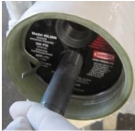
Removal of Head Assembly
