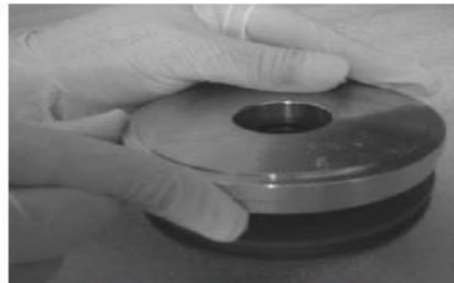
Installing Bearing Plate
