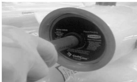
Installation of the End Plug Assembly into the vessel
