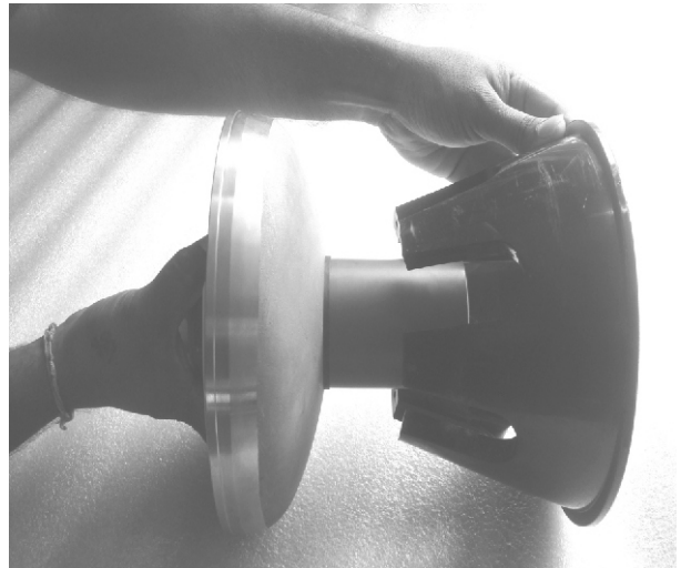
Installing Thrust Cone
