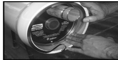
Installing Head Retaining ring
