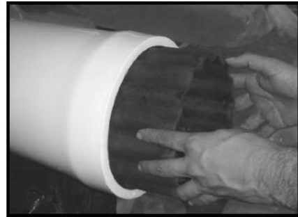
Installing Thrust Ring
