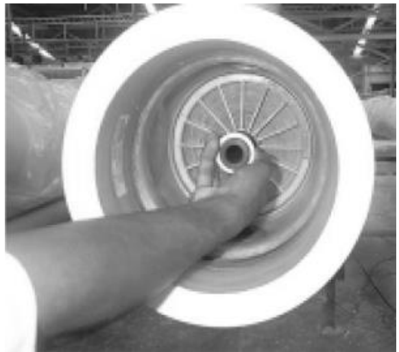
Vessel Shimming
