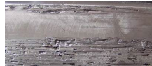
Abrasive wear on unprotected separating layer on outside
